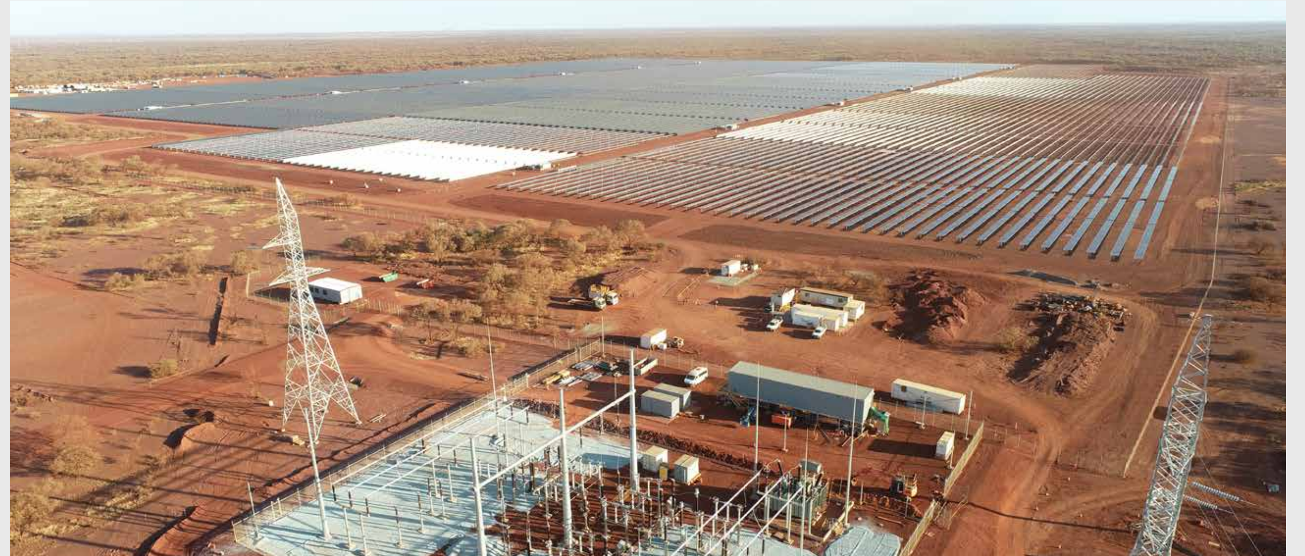
Image courtesy of Alinta Energy
